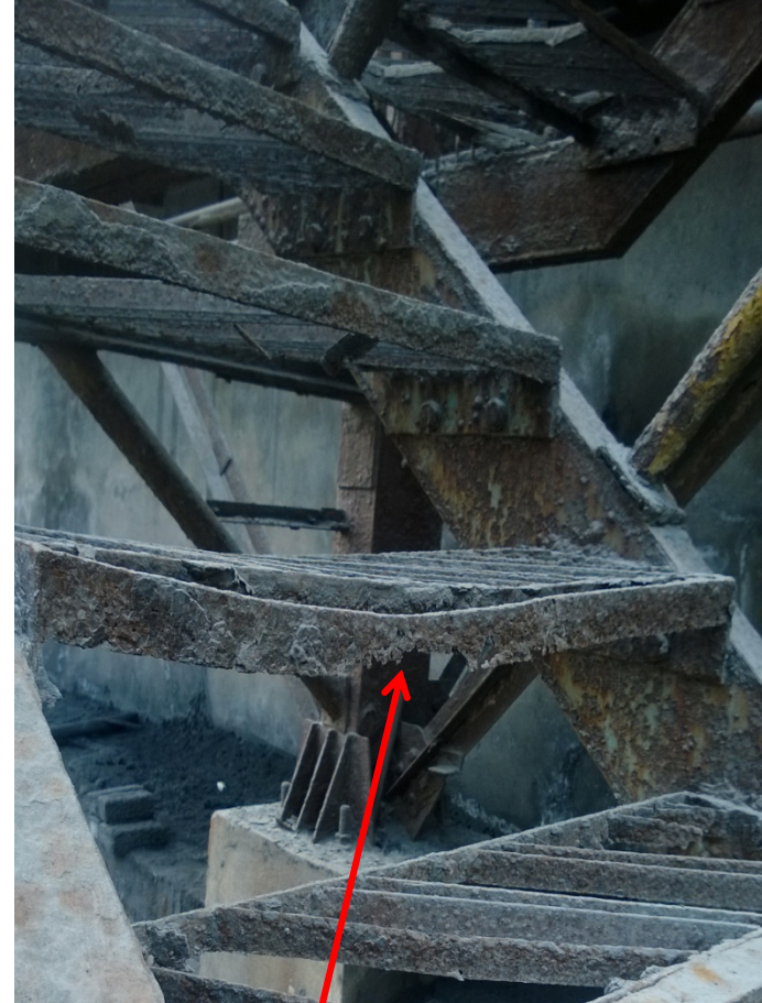
Significant chemical corrosion due to Na, K and Cl. Use of coconut fronds that collects a fair amount of NaCl that is usually administered as a nutrient is considered responsible
