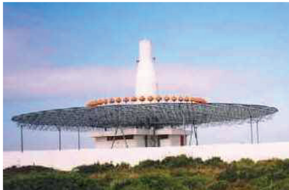
Figure 7.1.: The beacon is a combination of a Doppler VOR with a circle of orange balls and a TACAN identified by the cylinder in the centre. The ground station emits directional radio signals all around. The communication is line-of-sight dependent. Triangulation of position requires information from multiple stations
